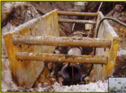
8' x 20' Trench Box on a job in Ft. Lauderdale, Florida.
