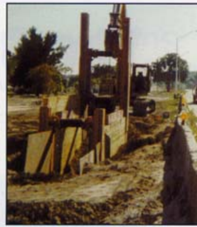
Installing the Krings Parallel system on Watson Island (Miami, Florida) for a french drain along side of the MacArthur Causeway between Miami and Miami Beach. 20' deep.
