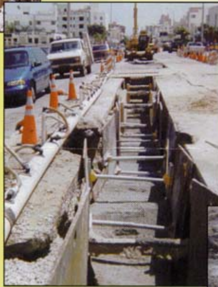
Hydraulic shores being used on a job in the middle of Collins Avenue on Miami Beach, Florida.
